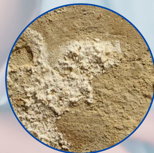
Efflorescence
